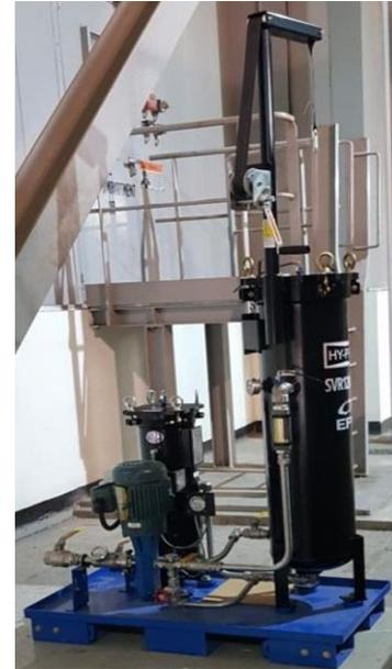
Moving ahead, the decision has been taken to install dedicated HYPRO SVR skids during 2018, on each of the GTs 1,2,3 as a permanent mount to enhance the reliability of Gas Turbines.
