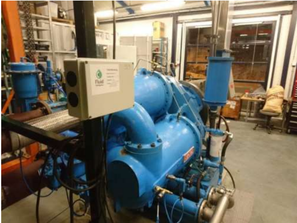
Lora Node installation next to compressor
